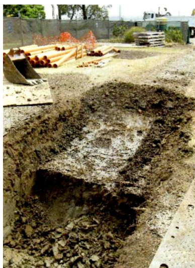
Top sediment layer of path revealed
