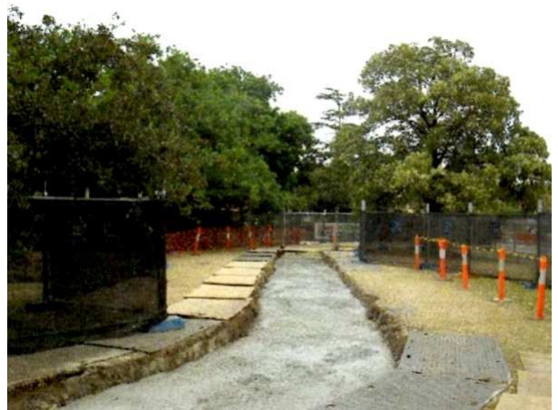
Trench containing power lines in a cement conduit
