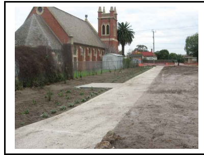
View of new development in progress
